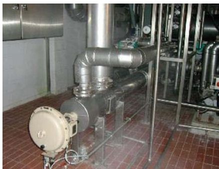
Figure 8-9: Thermal vapor re-compressor (TVR)
