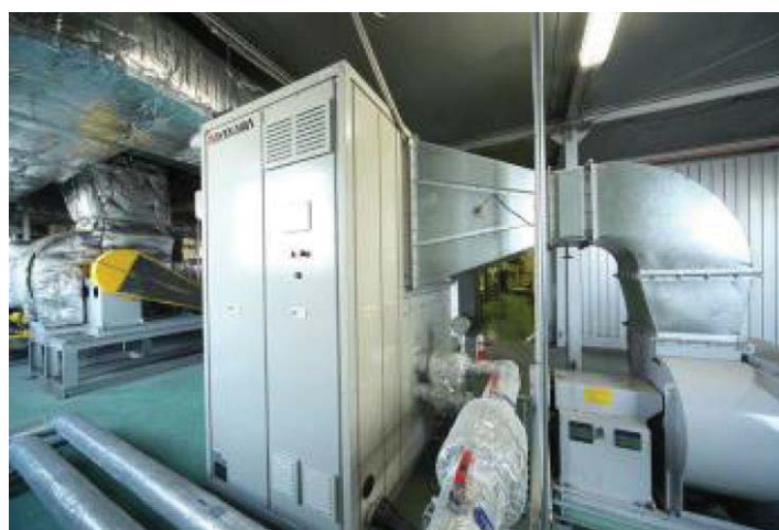
Figure 8-14: CO 2 heat pump air heater installation
