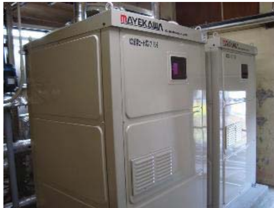
Figure 8-4: Simultaneous generation CO 2 heat pump of cold water and hot water
