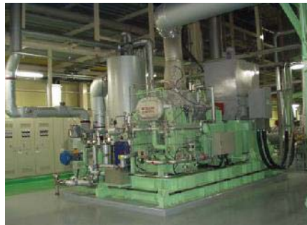
Figure 8-8: Mechanical vapor re-compressor (MVR)
