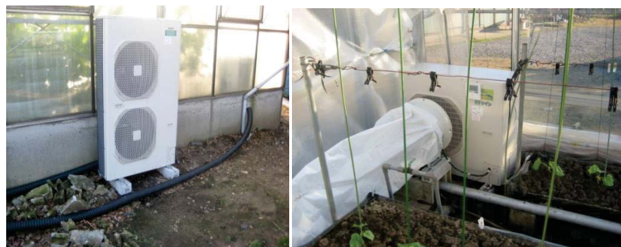
Figure 8-30: Heat pump outdoor unit (left), Heat pump indoor unit and circulating duct fan (right)
