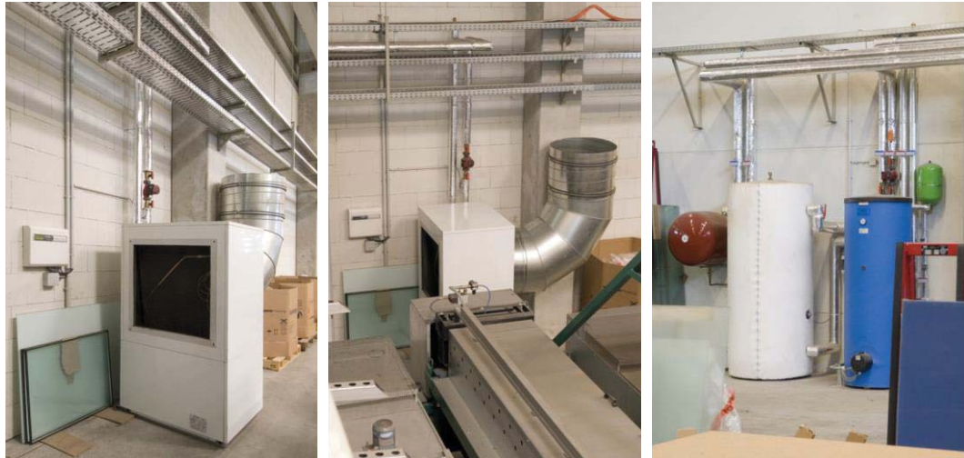
Figure 7-20: Air source heat pump situated directly next to the glass furnace /Dimplex 2012/
